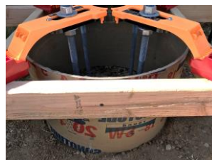
Room to trowel finish top of foundation base
