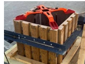
Setup for 24" Square Building Column
